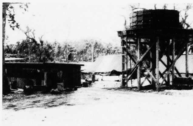
75th & 24th ASG Water Tower Shower Building
